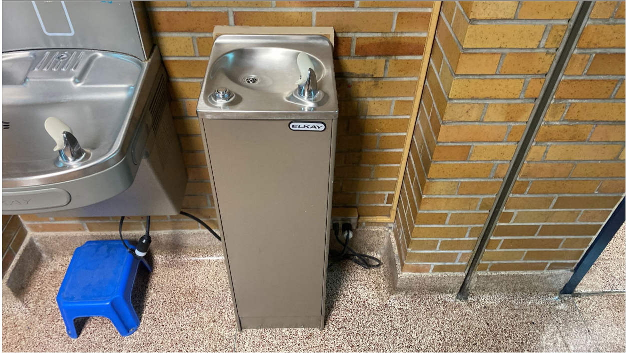
Taft-03: Hallway Across from Room 108, Water Cooler Fixture Removed from Service
